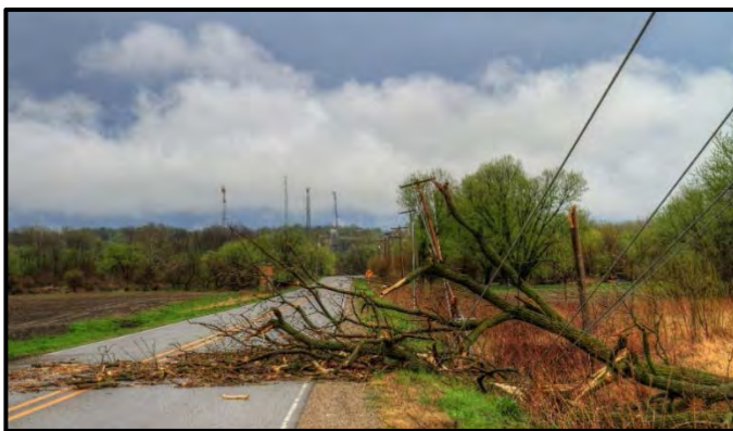
Figure 4.19. Straight-line winds toppled this dead tree into a power line and onto the adjacent county road.
