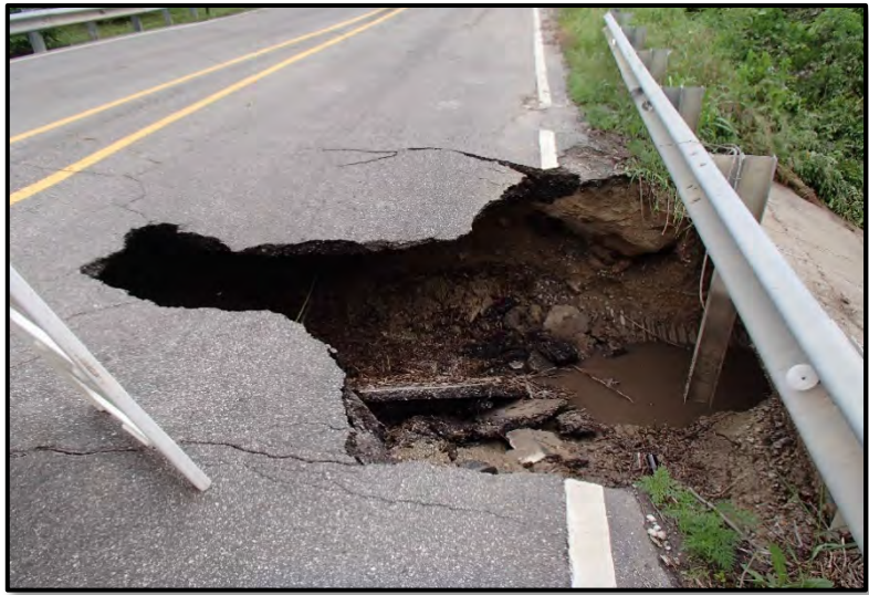
Figure 4.9. Scouring from a flash flood caused part of this roadway to collapse after a brief, but heavy rain storm.
