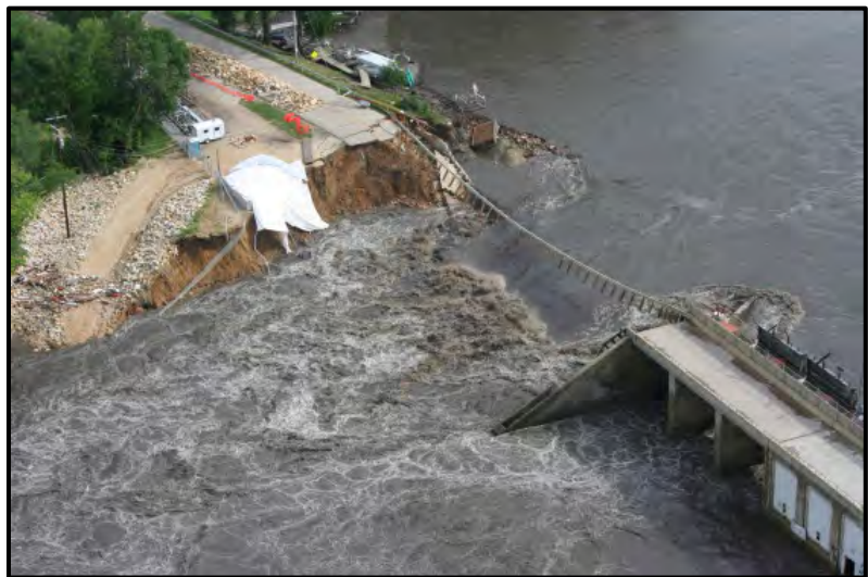
Figure 4.1. Dam Failure at Lake Delhi
