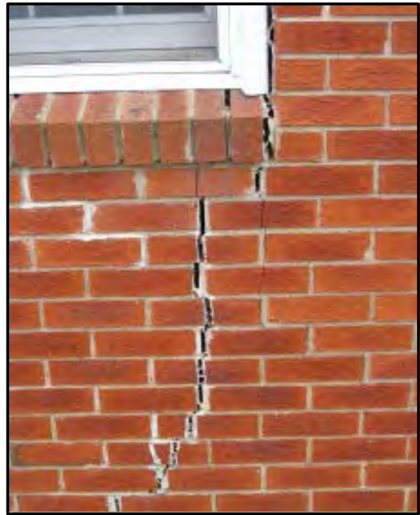
Figure 4.5. Cracked wall from a shifting foundation
